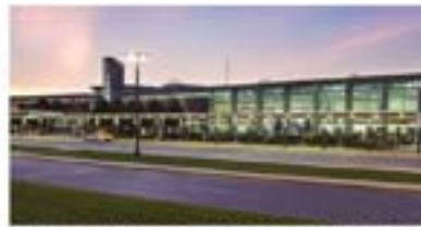
FAYETTEVILLE REGIONAL AIRPORT
